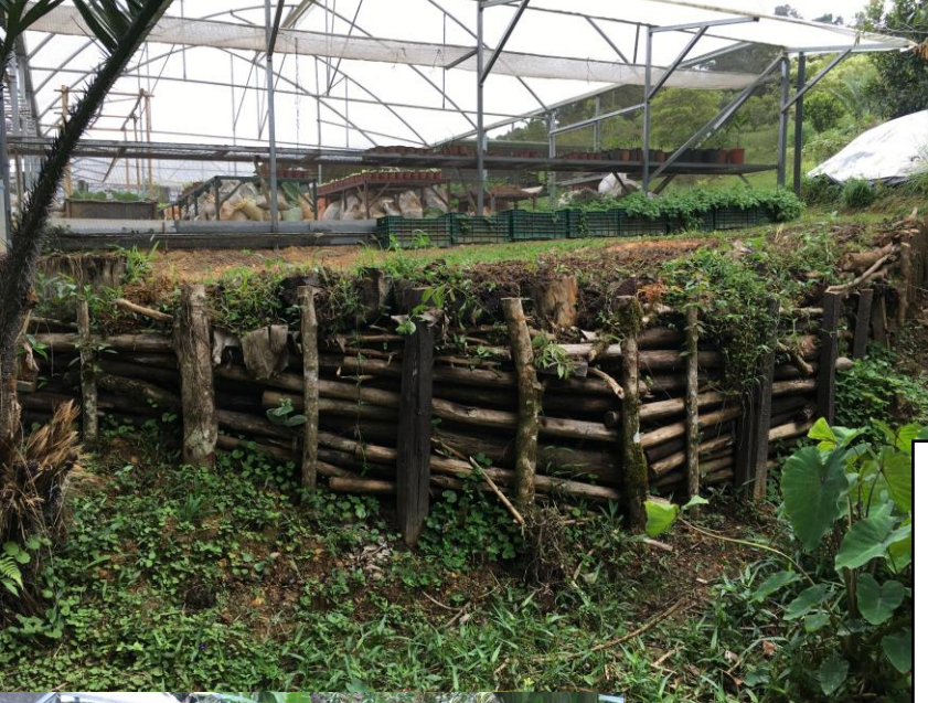
The south side of Al-Kauthar looking amazing after cutting back forest and building a retention to widen/level the space and help with water runoff. Improving drainages in Svarga and at the Spurana faucet.
